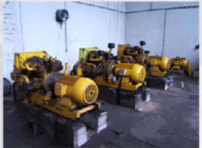
Name: Fagram – Smederevo Type: KS – 707 – 2 Manufacture: OOUR – Inzenjering Smederevo Capacity 25 m3/min Compressor ES 707 – 2 Work pressure 9 atm. Year of production 1981 Number of compressors: 4
