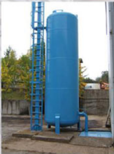
Name: Gas Reservoir Type: 118.29 Manufacture: Heroj – Srba Smederevo Work pressure 10 atm. Capacity 15 m quick Year of production 1981
